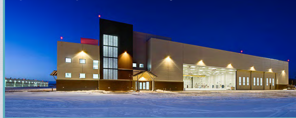
Squadron Operations Facility at JBER - Elmendorf
